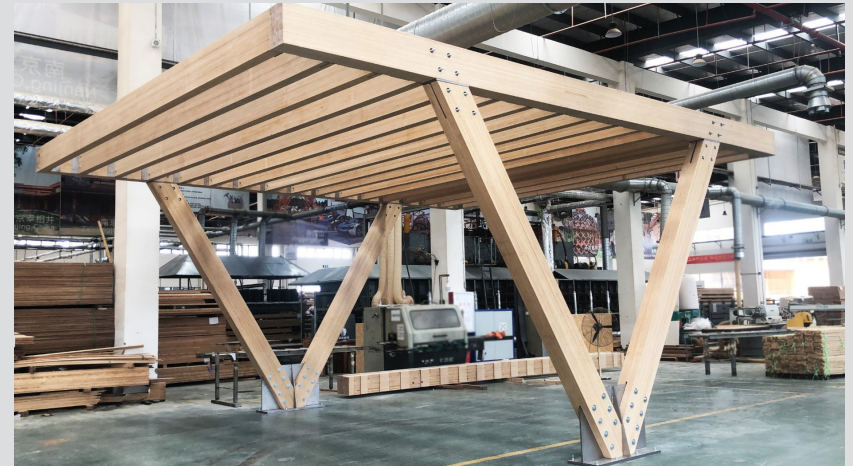
The structural bamboo canopy in the shop before installation.
